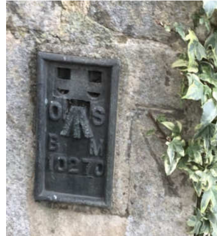
East view of the porch with the Victorian brass Bench Mark over the engraved stone Bench mark behind
